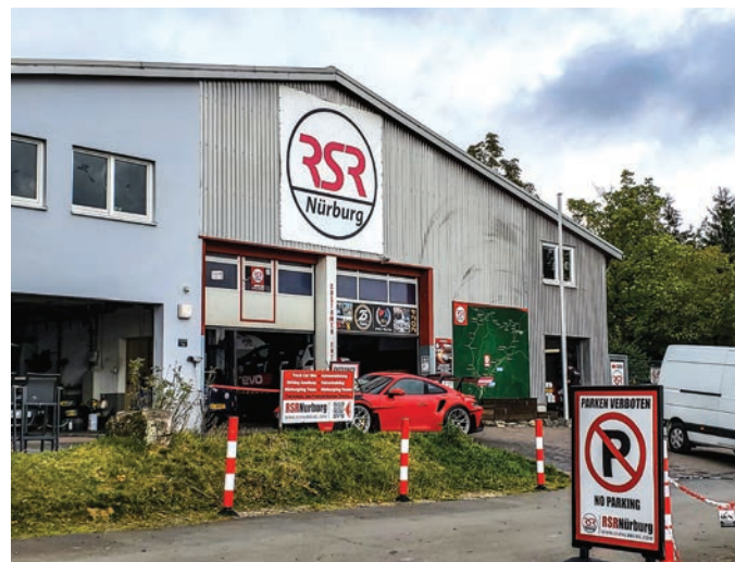
The RSR facilities at the Nürburgring, with service bays, classrooms, and administrative space.
