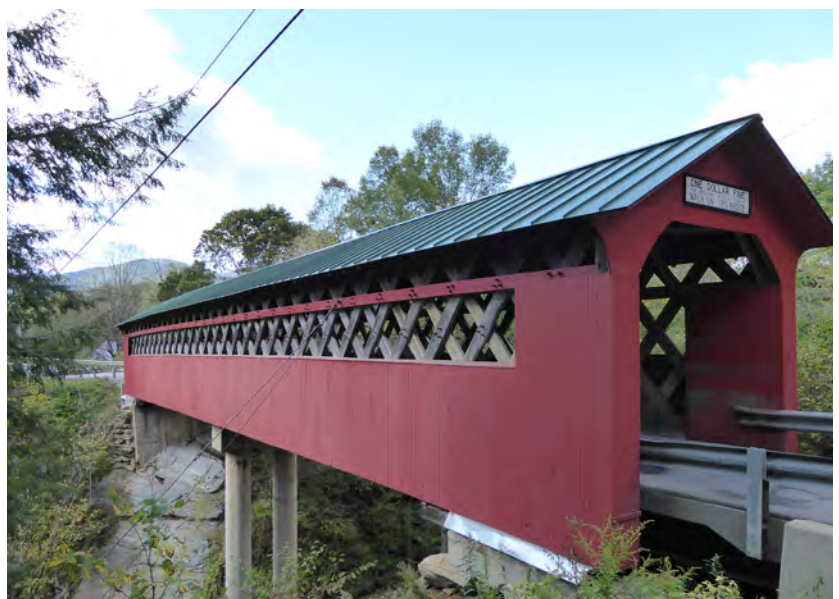
The Chiselville Bridge, Sunderland, VT
