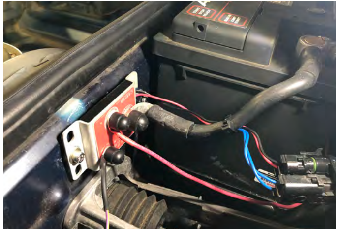
New electrical cutoff switch installed
