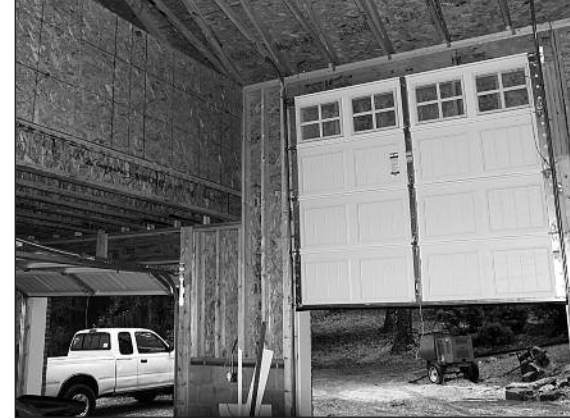
The “super bay” has an overhead door that allows for a lift. A storage room occupies part of the second level.
