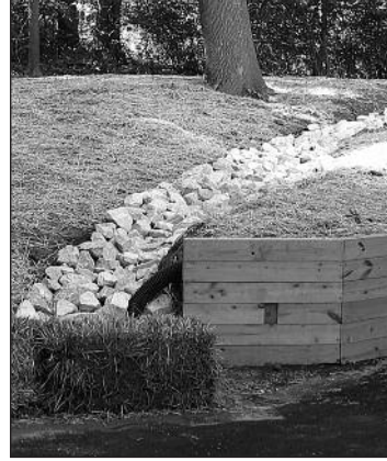
The finish line is in sight with landscaping, asphalt paving and provisions for drainage providing the finishing touches
