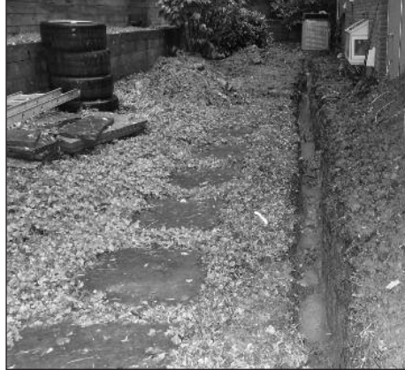
Bob had to dig this ditch by hand to install the electrical service. He has installed a lot of lights for illumination.
