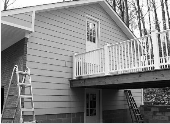
The garage is connected to the house by a breezeway and an overhead walkway.
