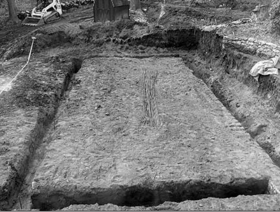
Construction began with footings, pouring concrete and installing rebar. Construction was hampered by rain throughout.
