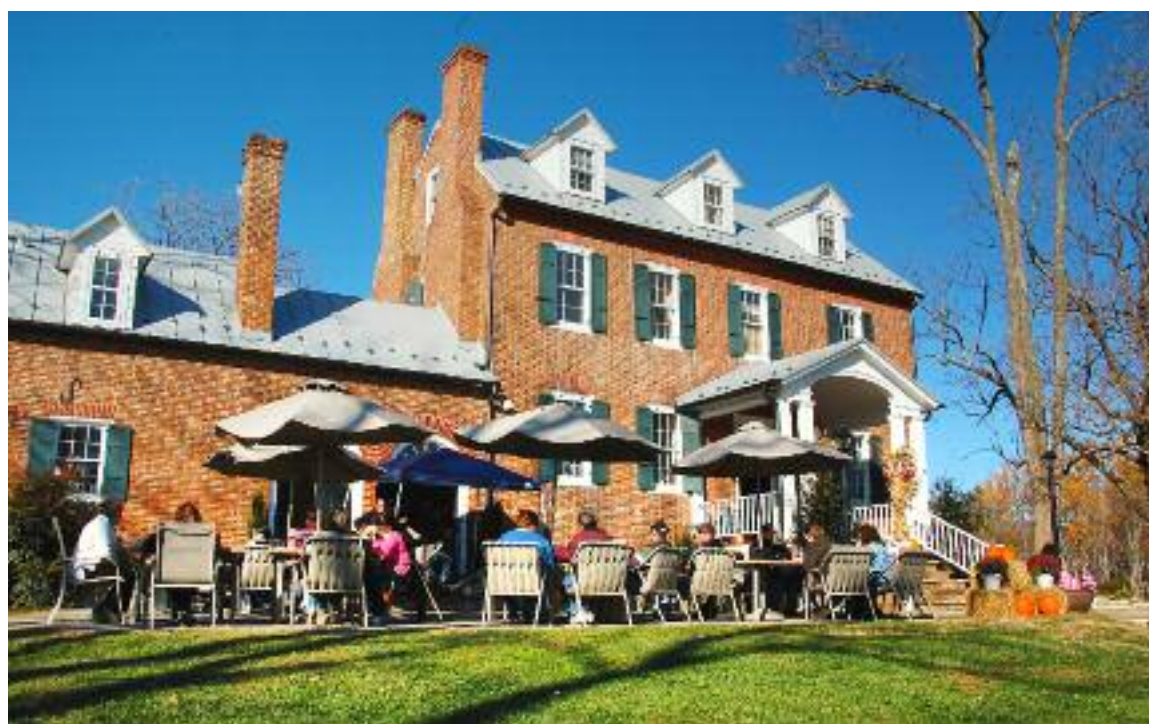
Photo by Richard Colella Above: La Grange is a restored three-and-a-half story red brick manor house built in the 1790s and recently renovated. A new winery building has been constructed on the winery grounds.
